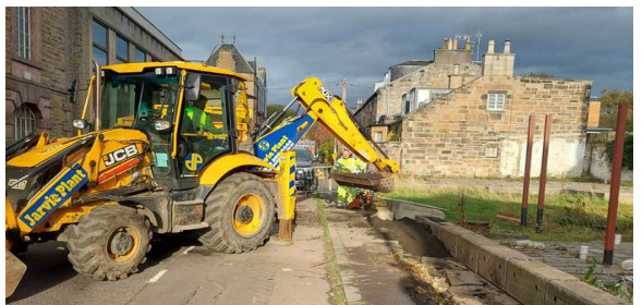
Workers in Upper Gray Street Thanks to City of Edinburgh Council
